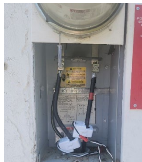
The primary side of the CT needs to be clamped on the Grid live line.
